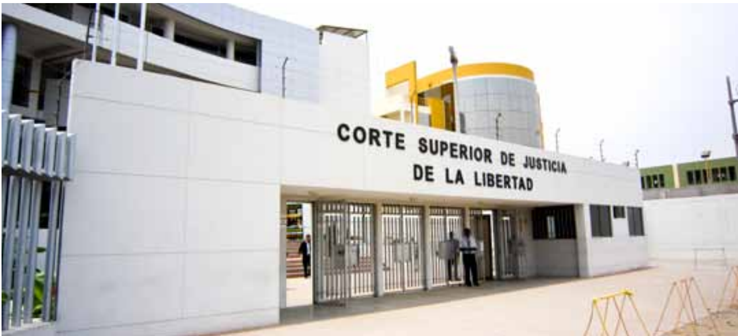
The High Court of the Peruvian district of La Libertad, part of an infrastructure project implemented by UNOPS on behalf of the Peruvian Judiciary and UNDP. Photo: UNOPS/Aida Arifo-Fernández
