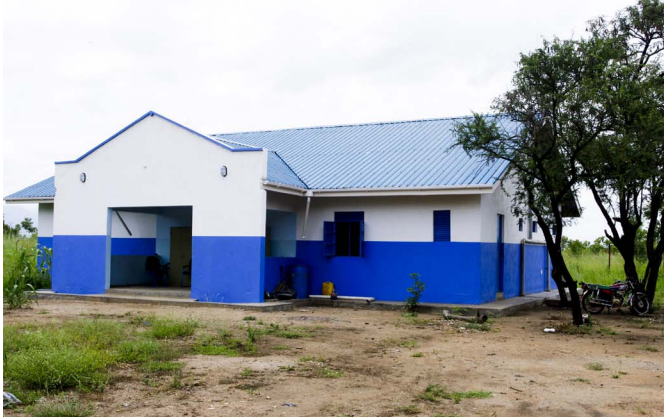
A police post in Eastern Equatoria, which has been credited with reducing cattle rustling and violent crime in the area, built by UNOPS on behalf of UNDP. Photo: UNOPS/Azusa Chiba
