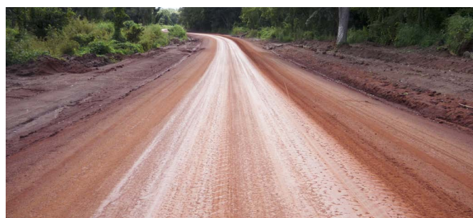
The change in conditions on the Diabio-Tambura road, after UNOPS implemented a USAID project. Photo: UNOPS
