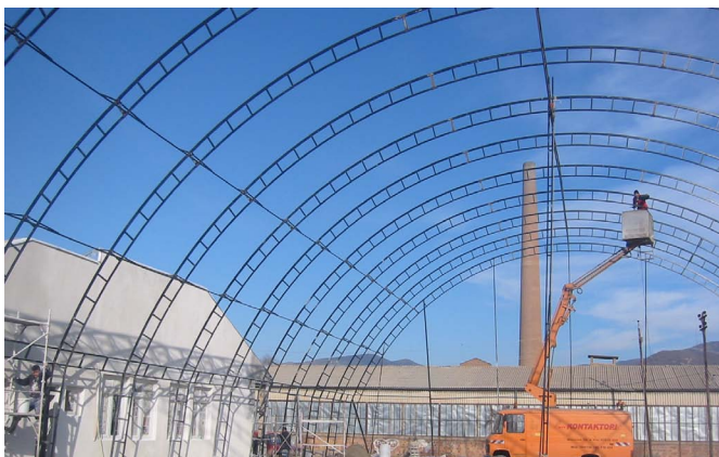
Construction of Sports Hall in Zvečan/ Zvečan Municipality
