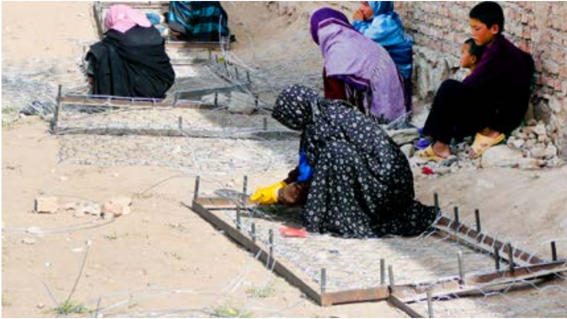
Women from the village of Jabraeel, Afghanistan make the wire baskets (gabions) needed to reinforce retaining walls and mitigate river flooding. The women, many of whom had never been employed before, learnt these new skills under a disaster preparedness project funded by the Government of Italy and implemented by UNOPS.
